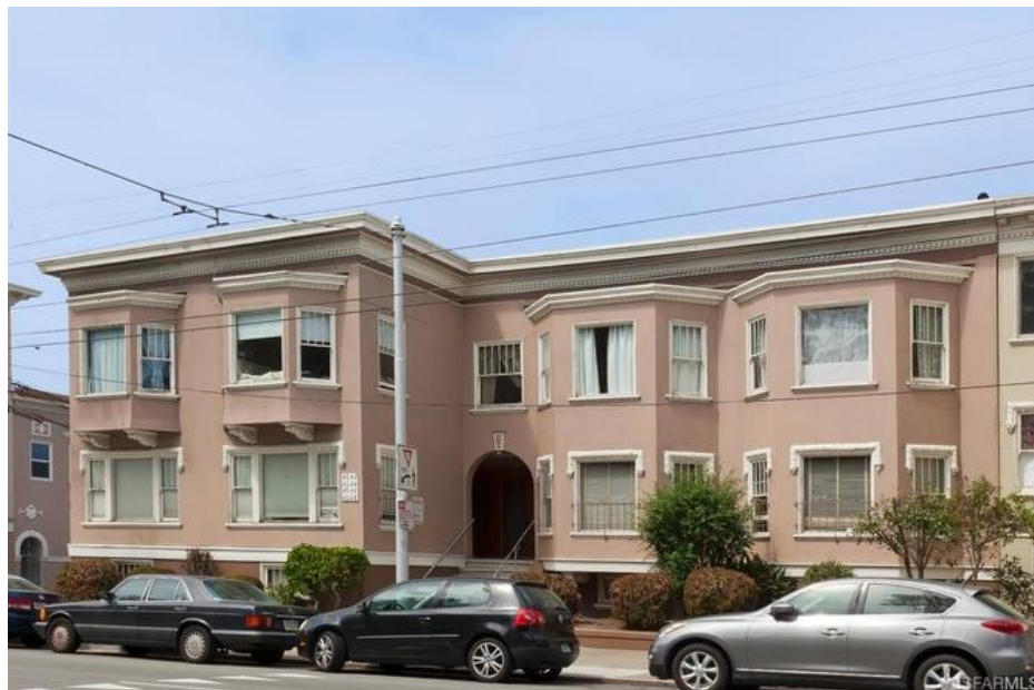
4042 Fulton Street - completed Feb 2018
