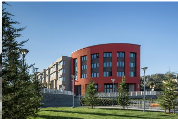
Hunters View Public Housing, post-transformation work
