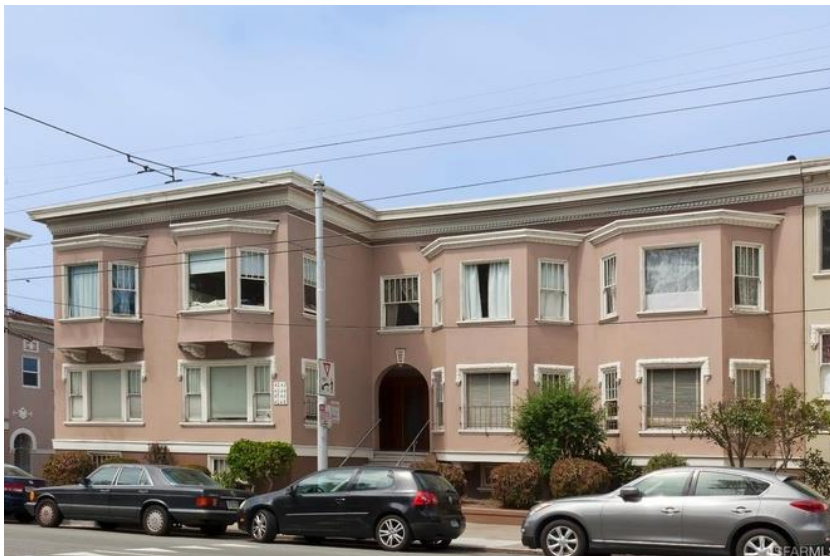
4042 Fulton Street - completed May 2018
