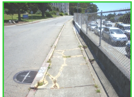
Narrow cracked sidewalks are greatly uneven, creating hazards
