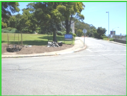
Poorly marked cross walks; curb cuts without yellow warning strips
