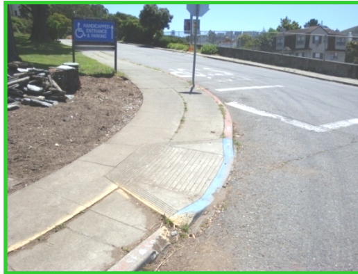
Deficient curb cuts; no crosswalk stripping
