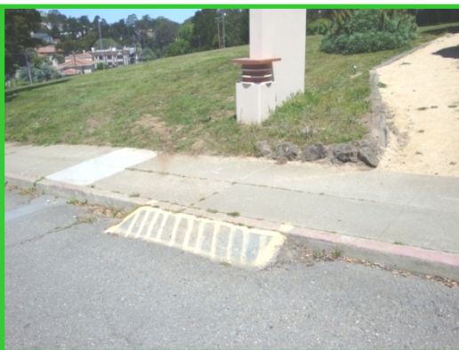
Makeshift "ramp" off sidewalk steep and dangerous
